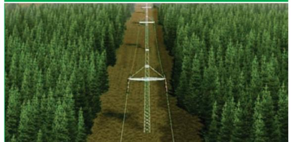
DC Corridor with one 500 kV bi-pole line for a total capacity of 3,000 MW
